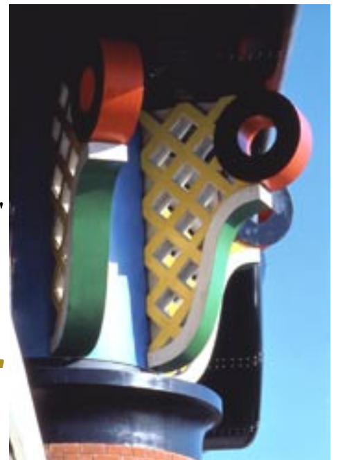
The 1980's Pumping Station in the Isle of Dogs remains a JOA rarity in that it is merely paint on white concrete. At least the substrate will not rust (and need scraping-down) before repainting.
